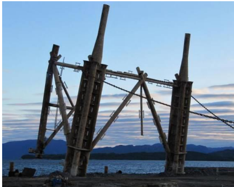
Figure 10.3 Removed Steel Jacket
